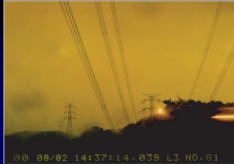
Flashover (direct lightning stroke to the middle phase conductor)
